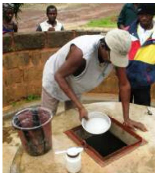
Fill ONE bucket of 10 litres with water. Pour TWO tablespoons of chlorine powder in this bucket. Mix it to dissolve the powder. Pour the chlorine solution into the well. Repeat this as many times as you need to drop spoons of chlorine into the well
