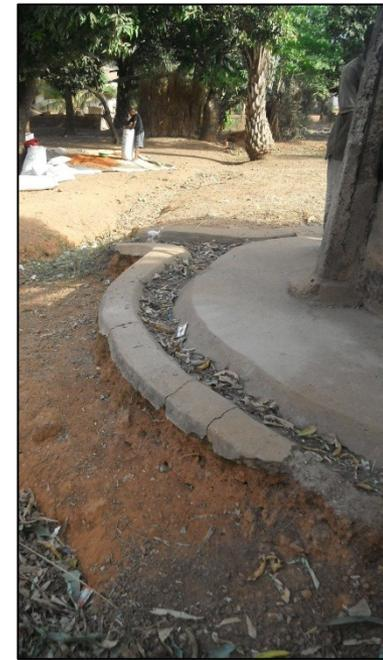
If the surface work was done with **no reinforcement** (soak away pit on the top) or with a **poor mixture** (apron on the right), after few months, several cracks will progressively appear.
