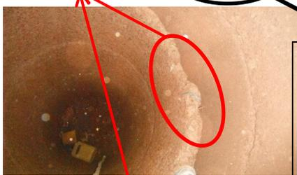
**Put stones at the bottom:** to avoid any clay to come into the well
